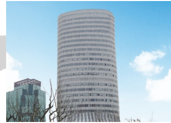
IMV CORPORATION Shanghai Representative Office
